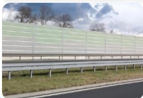
IMPLEMENTATION OF ROAD AND RAILWAY SCREENS
