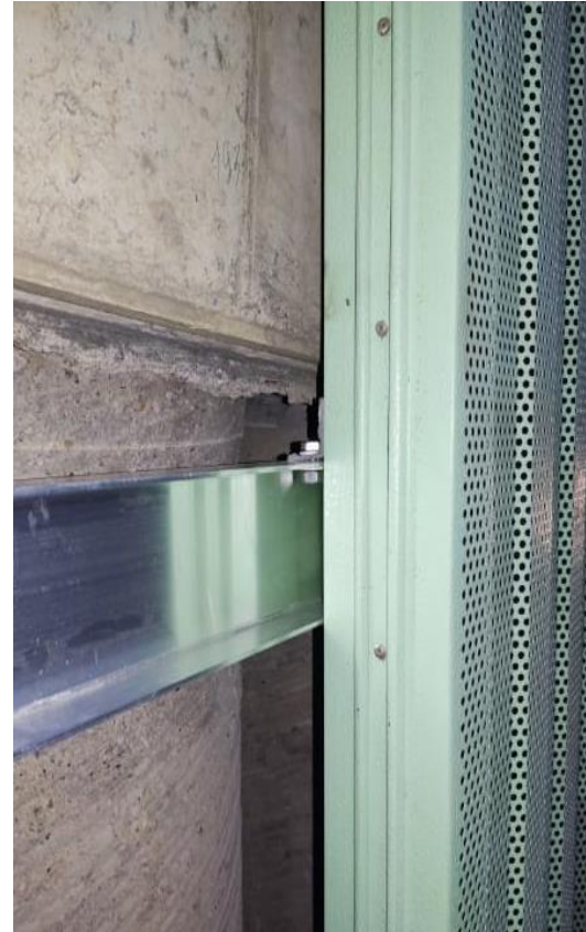
Photo 7;8. Execution of the substructure for the palisade facing at the implementation stage for the task titled "Construction of the bypass of the city of Wałbrzych along national road No. 35 from km 2+350 to km 8+250"
