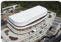
ACOUSTIC ROOF SCREENS
