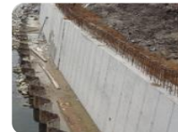
CONSTRUCTION OF SHEET WALLS REINFORCED WITH CAP
