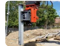
CONSTRUCTION OF FOUNDATIONS FOR ACOUSTIC SCREENS USING DRIVEN STEEL PILE TECHNOLOGY
