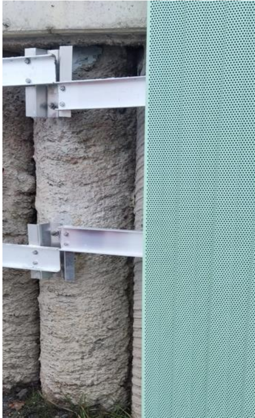
Photo 7;8. Execution of the substructure for the palisade facing at the implementation stage for the task titled "Construction of the bypass of the city of Wałbrzych along national road No. 35 from km 2+350 to km 8+250"
